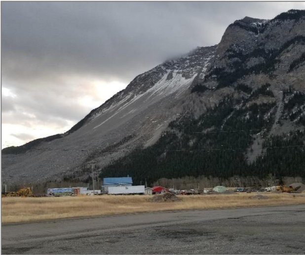
FIGURE 27 - FRANK INDUSTRIAL PARK
