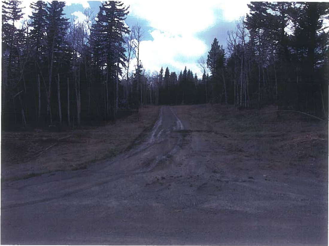
Existing Access Road
