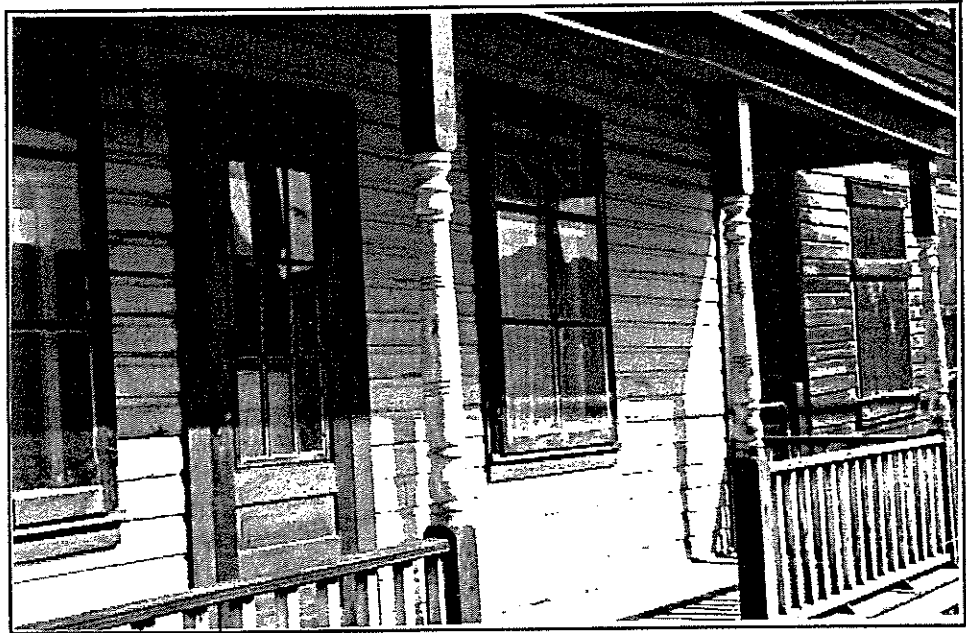
Fig. 112 Coleman, 1990 Verandah running full length of house front facade.
