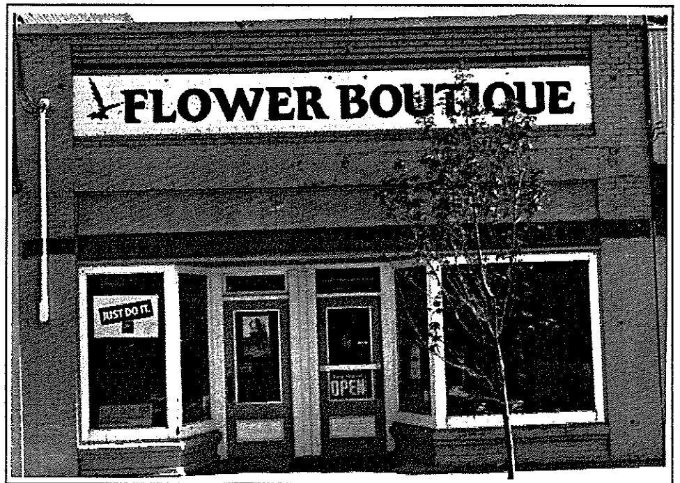
Fig. 52 Blairmore, 1990 Brick boomtown style (1905) building with a now rare double storefront on a 25 foot lot.
