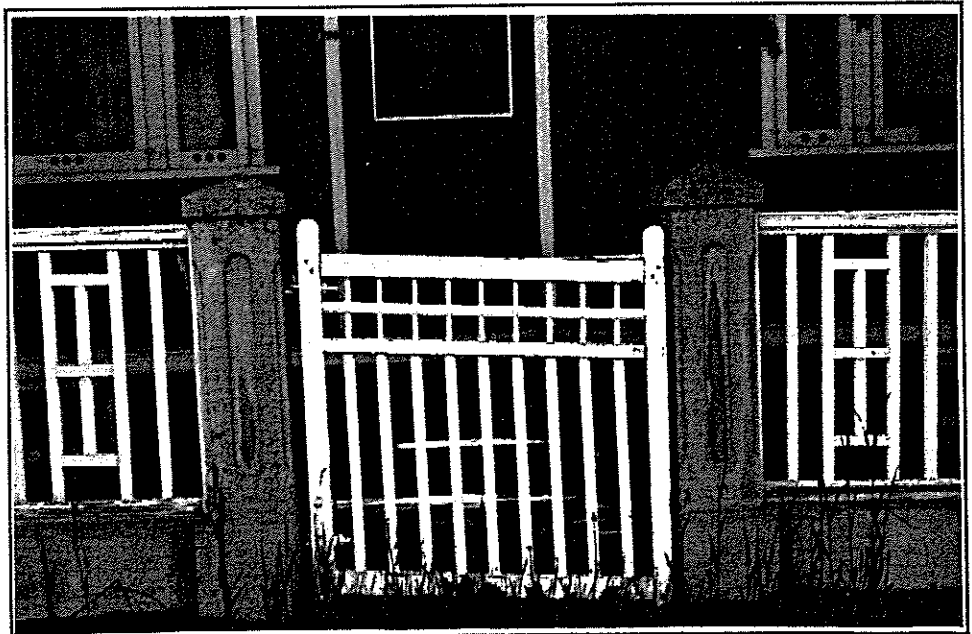
Fig. 119 Blairmore, 1990 Cast stone posts with decorative geometric patterns of rails and pickets.
