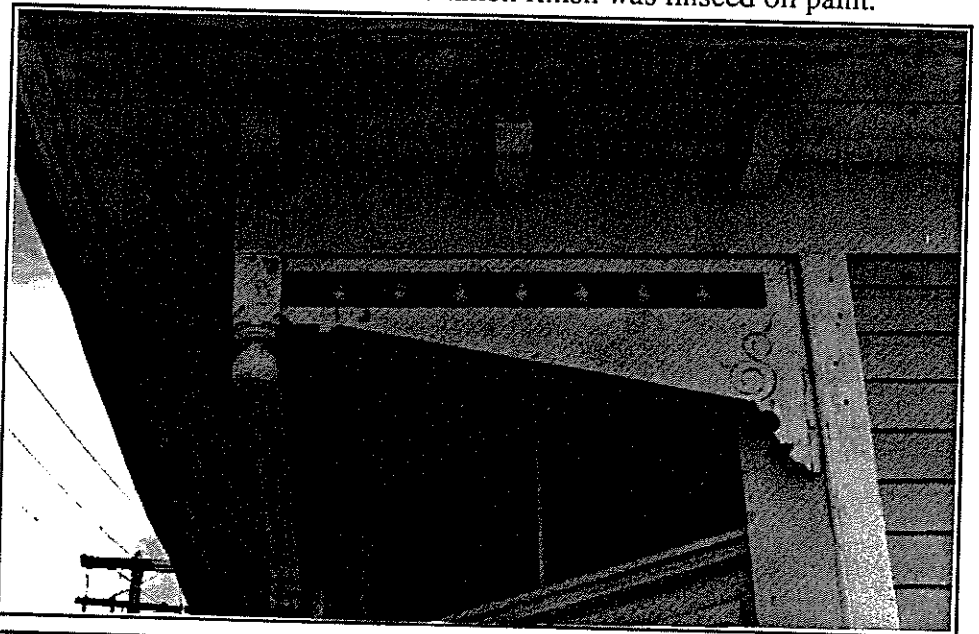
Fig. 64 Coleman, 1990 Decorative wood brackets at entrance of The International Coal and Coke Com- pany (1904)
