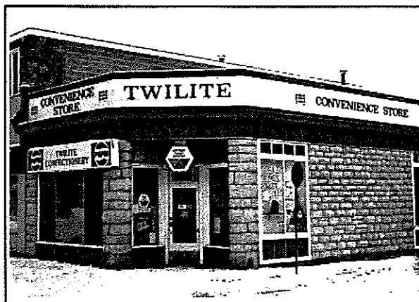
Fig. 143 Blairmore, 1990 Twilite Confectionary Replacement of the cornice and cleaning paint from the limestone returned this building to its earlier appearance.
