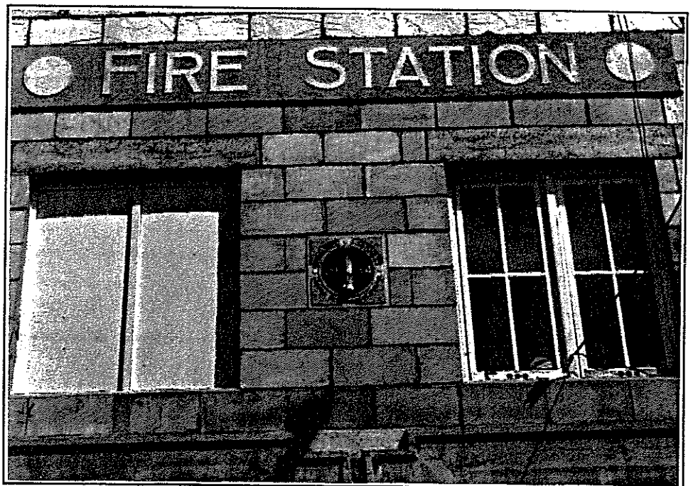
Fig. 73 Coleman, 1990 Fire Station (1907/134). Detail of cast stone facade with stucco signband.
