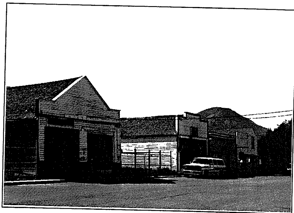
Fig. 77 Hillcrest 1990 Similarly scaled Main Street buildings.
