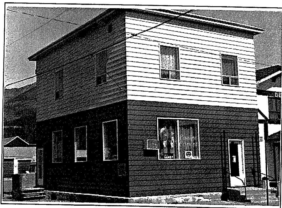
Fig. 25 Bellvue, 1990 Former Royal Bank (1911) retrofitted with vinyl siding.
