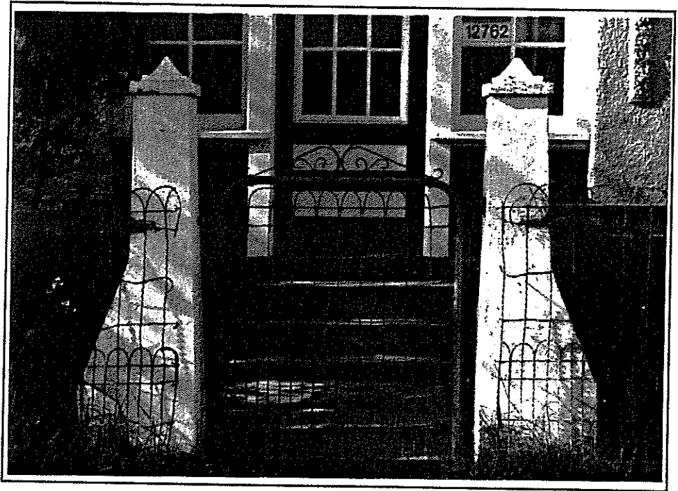
Fig. 190 Blairmore, 1990 Cast stone posts and wire fencing were a traditional material of the historic period
