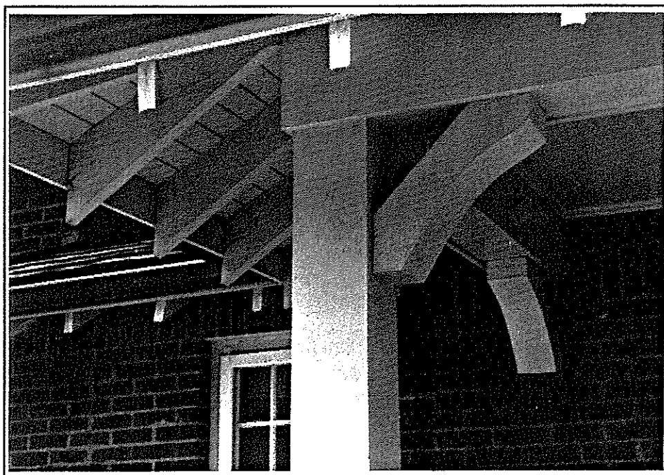
Fig. 166 Blairmore, 1990 AGT Block Frequently maintained wooden brackets.
