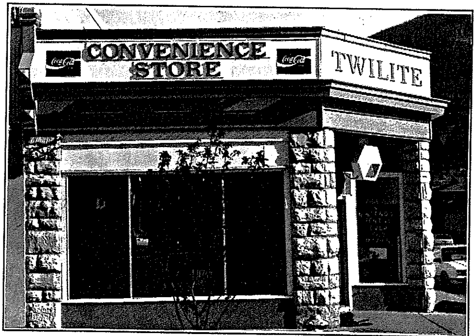
Fig. 151 Blairmore, 1990 The Twilite Confectionery, with cornice replaced.
