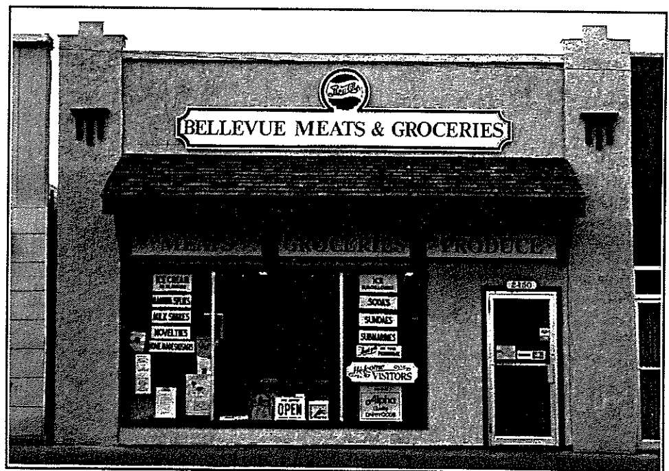
Fig. 156 Bellvue, 1988 Bellevue Meats and Groceries The metal siding was removed from the storefront, and the facade was re-stuccoed. A fixed canopy, that echoed the design of a canopy on the same street, was added to protect this south facing facade from internal heat build up.
