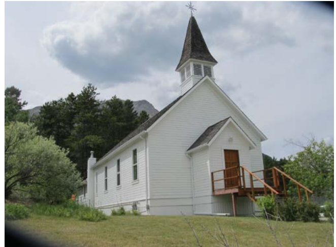
Figure 64: Hillcrest United Church, Hillcrest, 2015.
