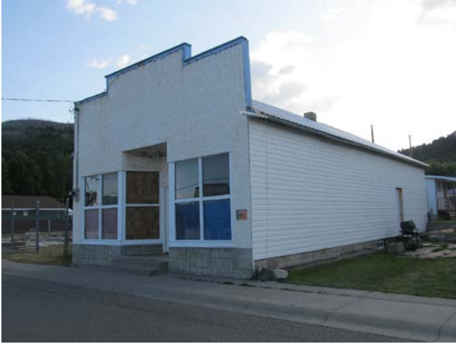
Figure 61: Hillcrest Trading Company building, Hillcrest, 2015.
