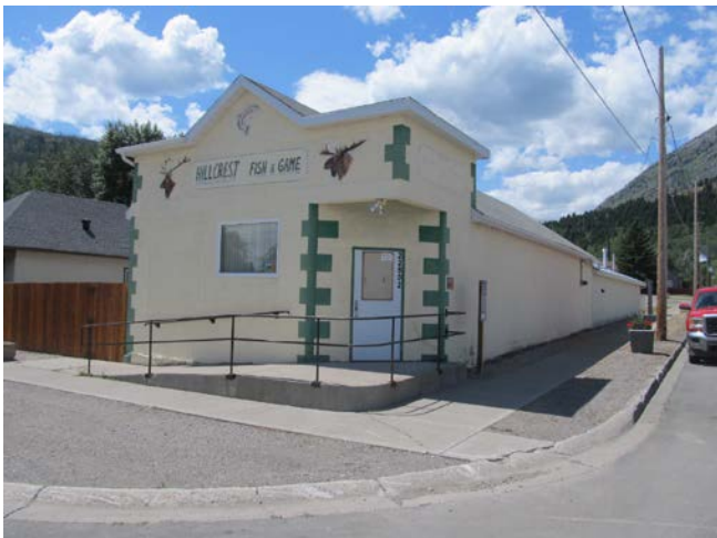
Figure 62: New Canada Café building, Hillcrest, 2015.
