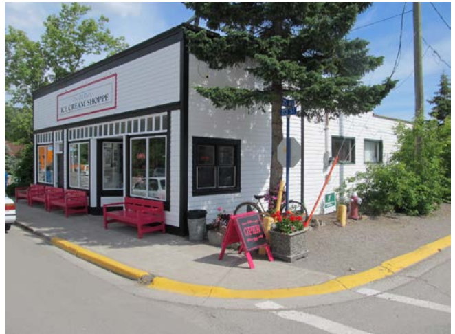
Figure 29: Emmerson Building, Bellevue, 2015.
