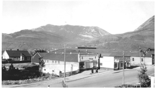
Figure 28: Emerson Blais Building. Crowsnest Pass Museum and Archives.
