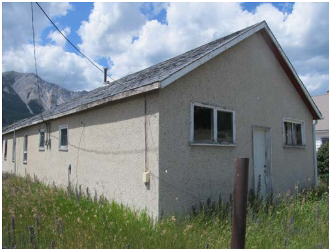
Figure 16: West Canadian Collieries Boarding House, Bellevue, 2015.
