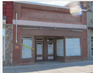
Figure 47: Kubik's Meats and Groceries building as it exists in 2014.
