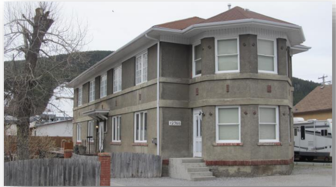
Figure 29: The Greenhill Apartments as it stands today in 2014.
